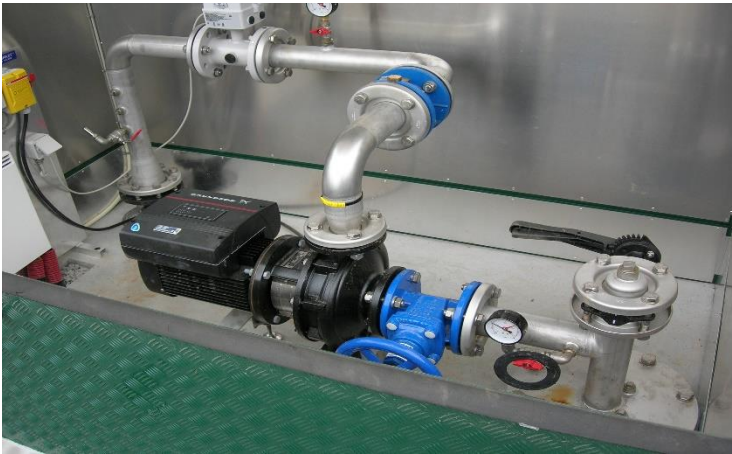
Pumpe m.m. i ny boring
